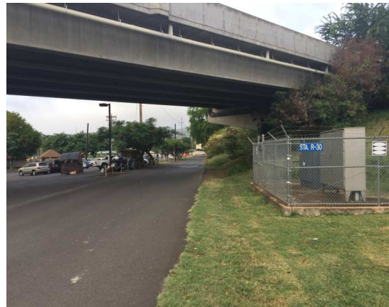
View of Existing Arizona Memorial Drive
