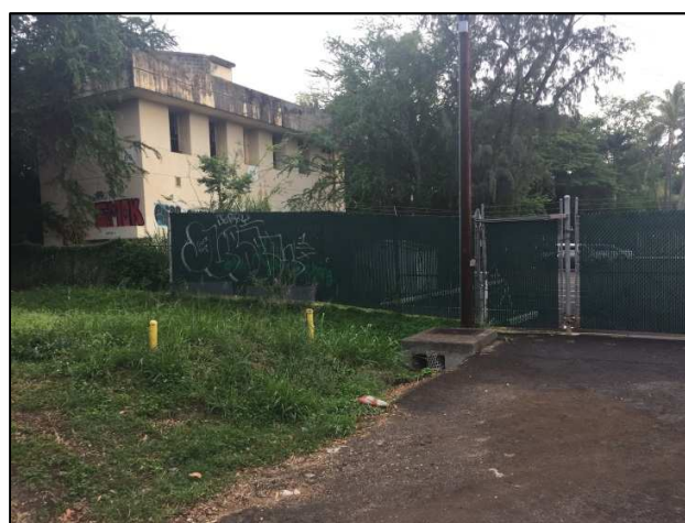
The existing PHHT ends at a fence near the Bombproof Switch Station on one end and the Admiral's Boathouse on the other.
