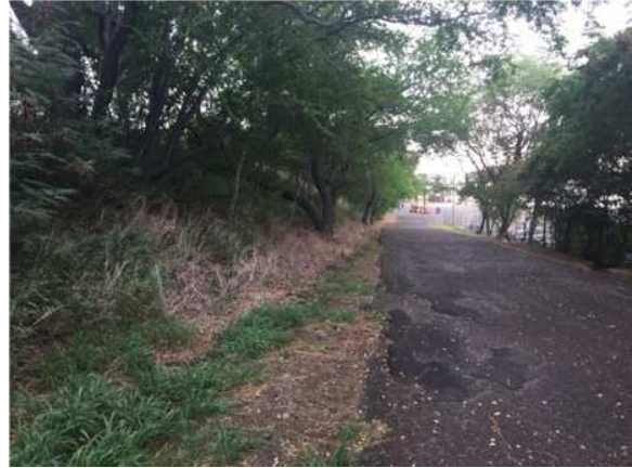
View of Existing Richardson Road
