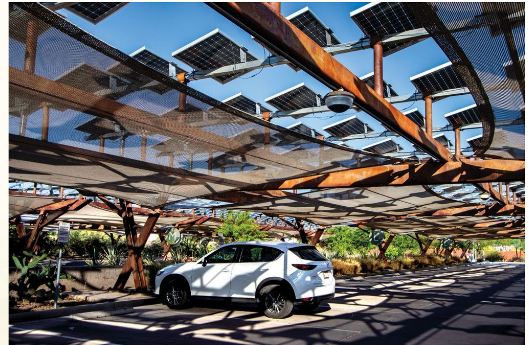
Location & Source: Springs Preserve Las Vegas
